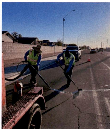
Crack Seal
