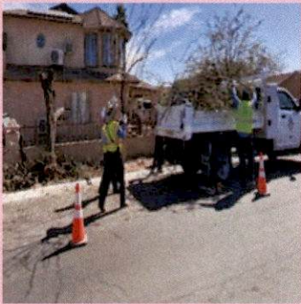
Assist Public Works in removing a tree in the right-of-way.
