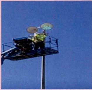
Replacing burned light bulbs in F2 and F3.
