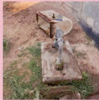
Broken leaking backflows were repaired.
