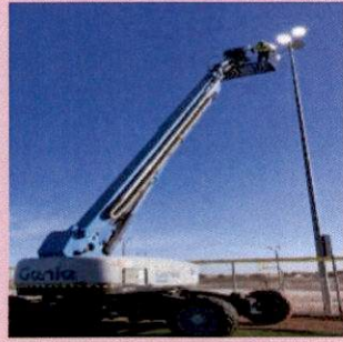
Replacing burned light bulbs in F2 and F3.
